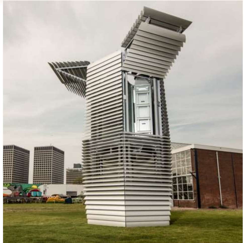
Smog Free Tower – Roosegaarde – ionization of PM © Roosegaarde
