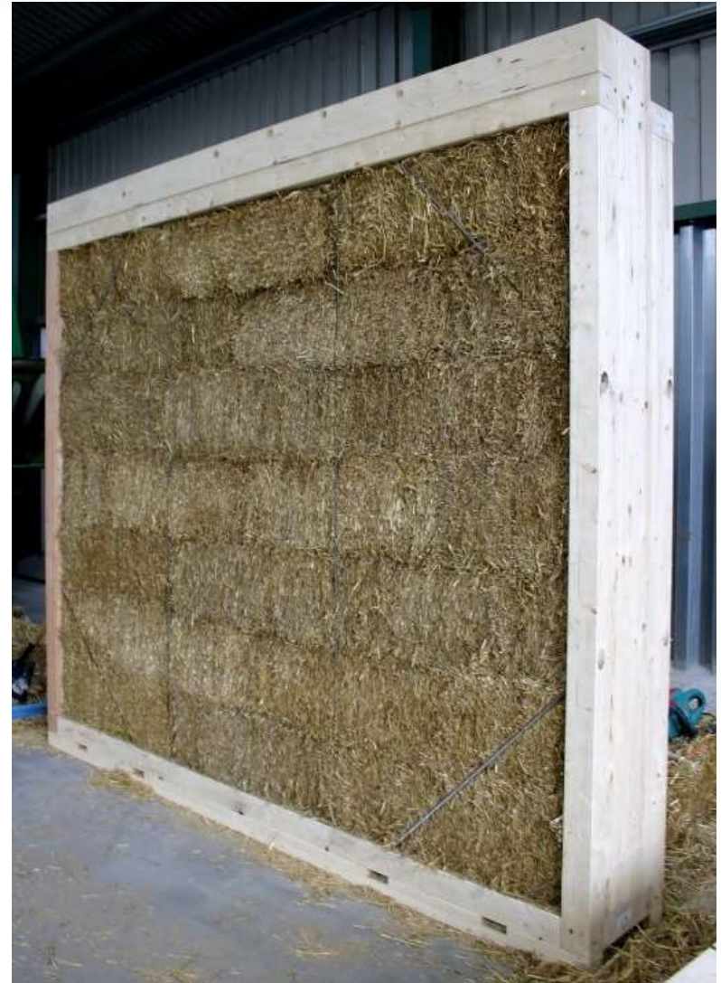
Straw insulation - Modcell
